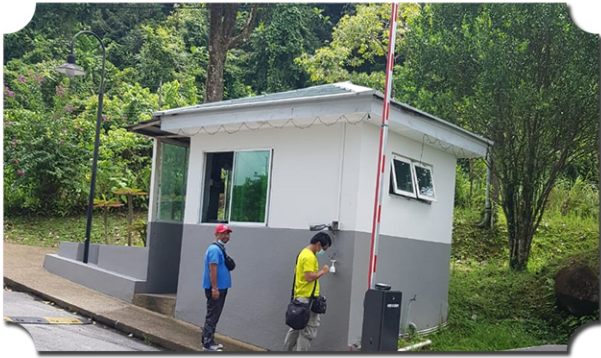
BARRIER GATE SYSTEM
